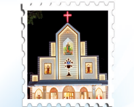
The Renovated St. Thomas Church, Chandrapur (23.04.2023)
